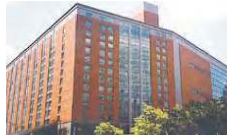
Embassy Suites at Battery Park City — New York, NY
